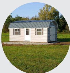
Build On Site *Varies By District
